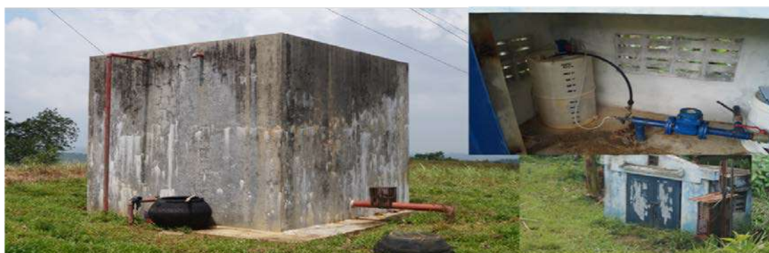
Dawis Pumping Station and Reservoir
