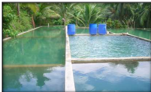
Manampa Sedimentation and Filtration
