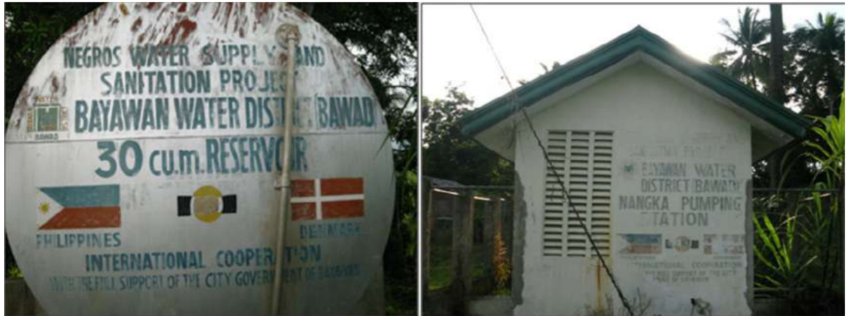
Figure 10 Nangka Pumping Station and 30 cum Reservoir
