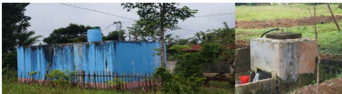
Ali-is Spring Box and Reservoir.
